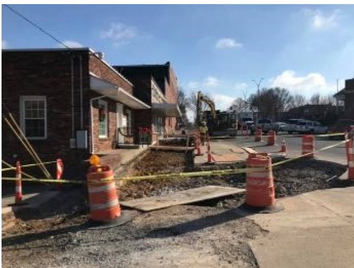
Streetscape work beginning in downtown Scottsville!
